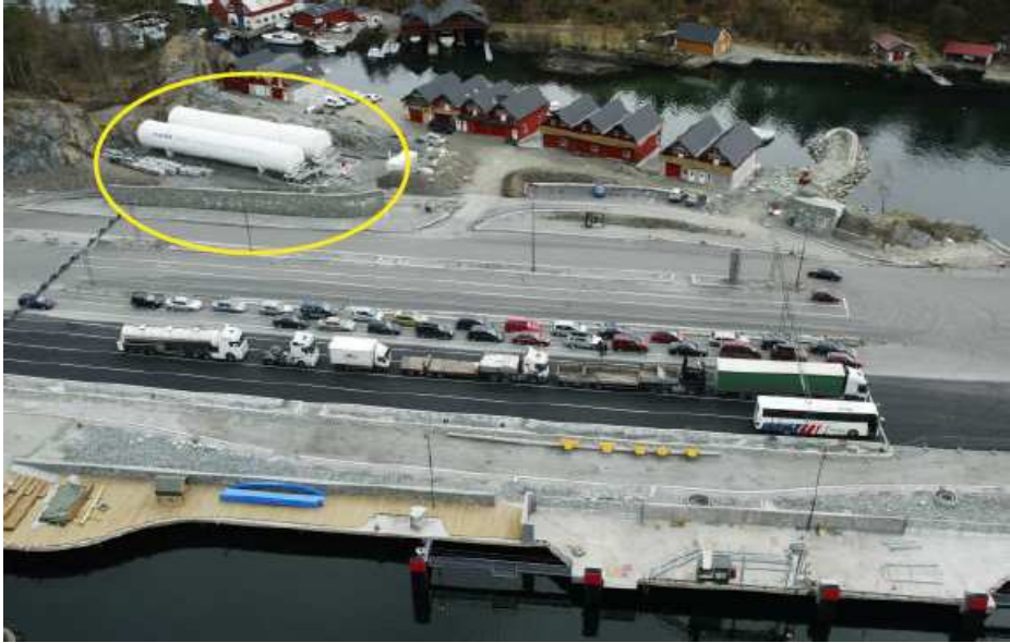
Figure 6. The LNG terminal for bunkering purpose at the Halhjem ferry quay Source: The MAGALOG project- LNG fuelled shipping in the Baltic Sea - presentation
